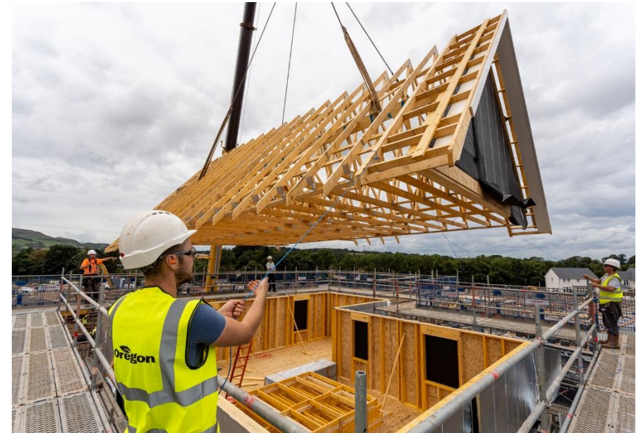
Oregon timber frame installation
