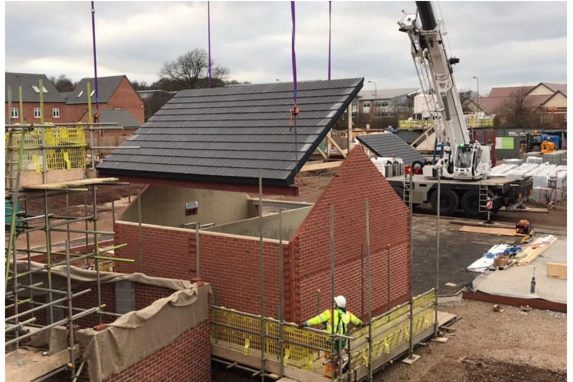
Offsite concrete garage trial in Nottingham
